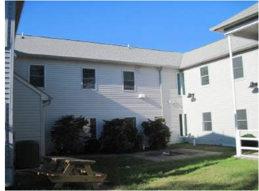
Building B contains a commercial kitchen, lounge area, laundry, computer room, and 10 apartments.
